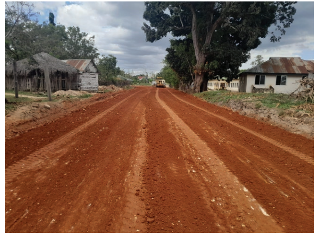
Work on 32km Utete – Kingupira Road, Rufiji, Pwani
