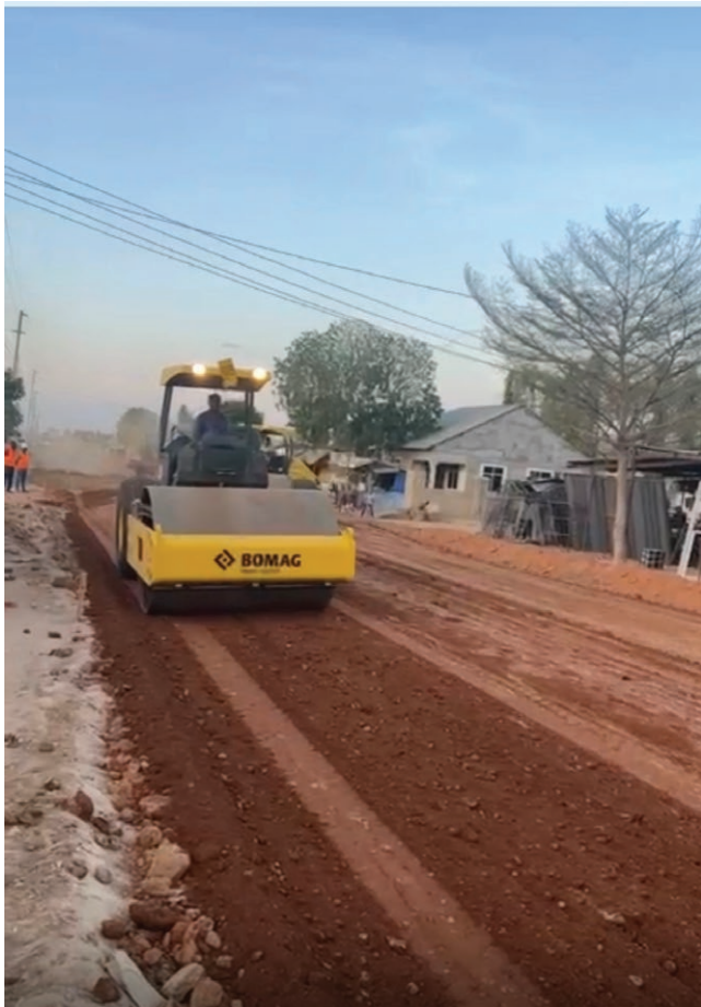
Compacting the base surface after the soil has been mixed with
