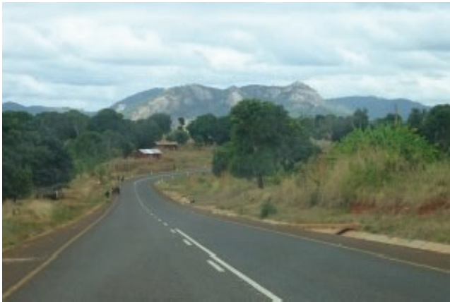
Section of 267km Tunduru – Songea Road, 9th June 2016 [Photo: American couple]
